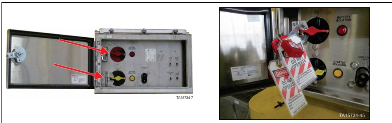
GEN 2 Battery Isolation Box – Battery isolation switch in OFF position with locks in place
