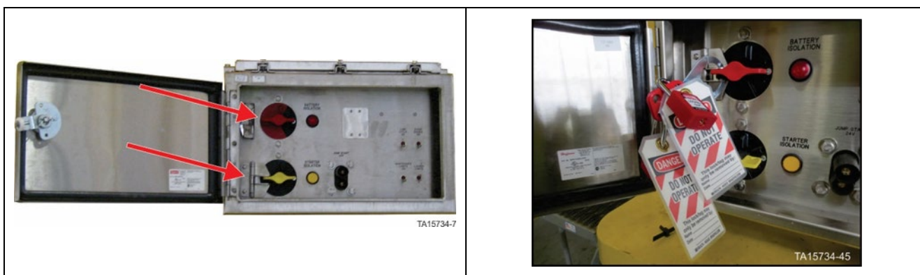
GEN 2 Battery Isolation Box – Battery isolation switch in OFF position with locks in place
